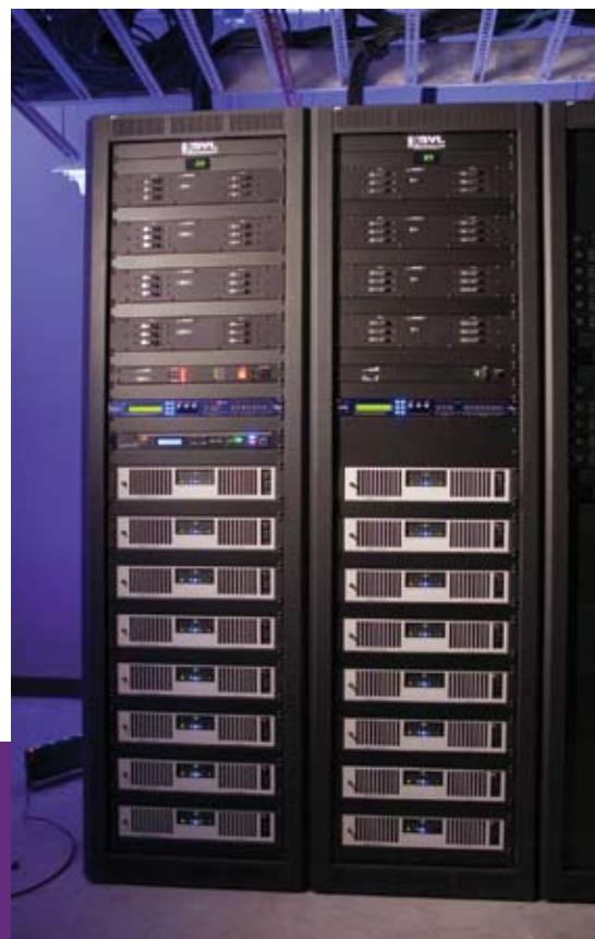
Lab.gruppen audio amplifiers power the church's SLS loudspeakers; Shure wireless receivers share rack space in the amp room.
